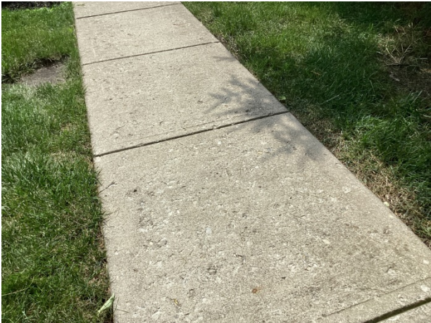
Sidewalk spall
