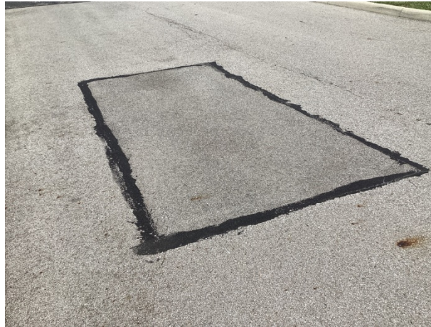
Previous patching repair
