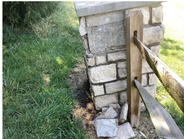
Significant masonry damage
