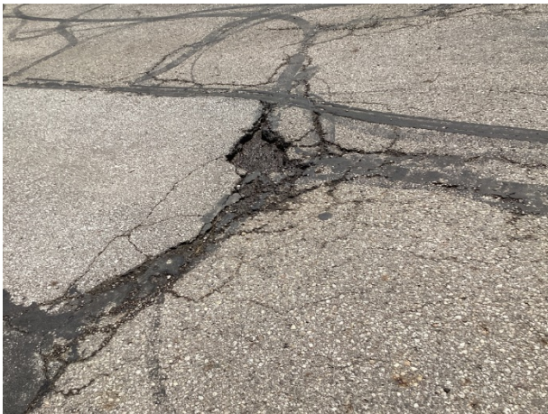
Pothole and surface deterioration
