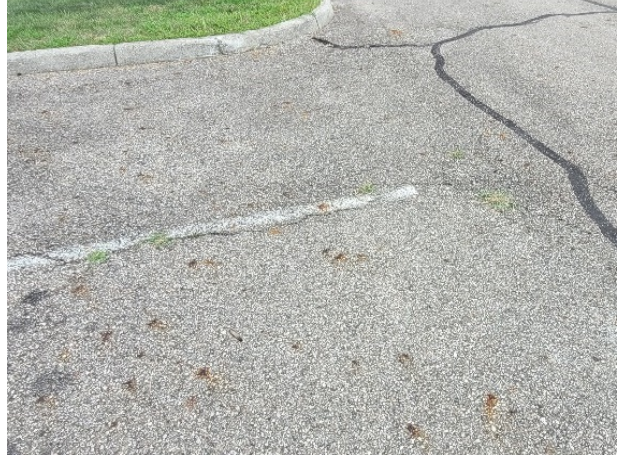
Settlement and pavement cracks
