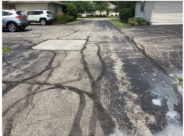
Phase Two access drive overview, note surface wear, previous patching and deterioration
