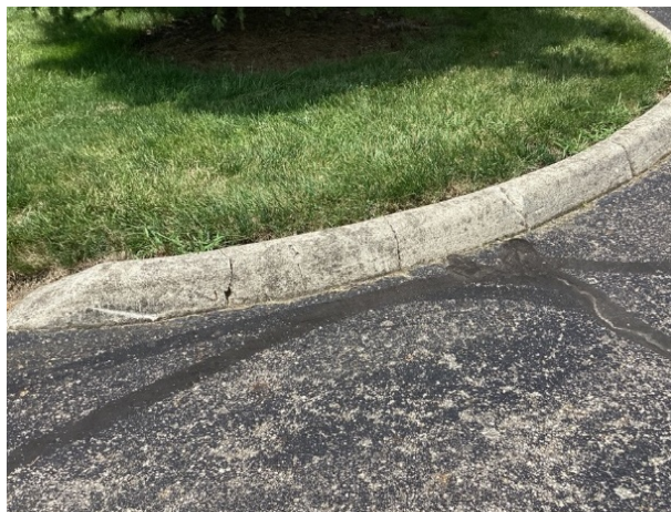
Concrete cracks
