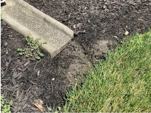
Granular loss, shown at Building 7
