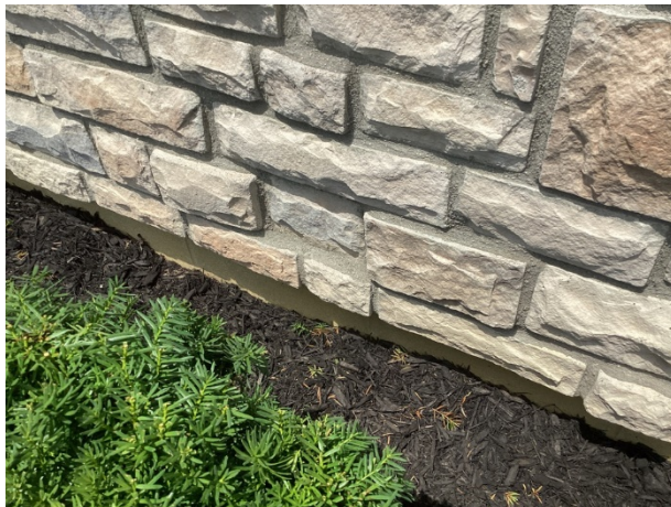
Apparent missing masonry
