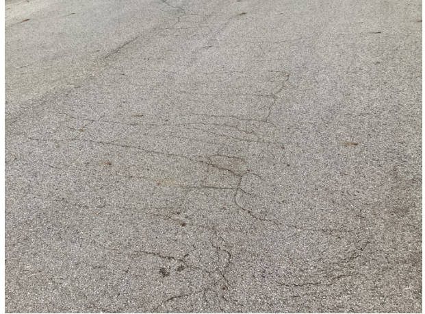
Pavement cracks
