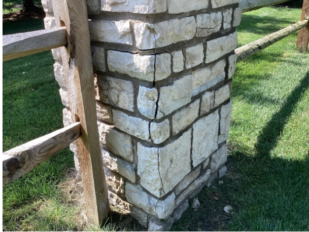
Masonry cracks
