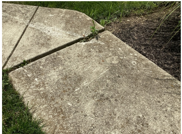
Concrete deterioration and organic growth
