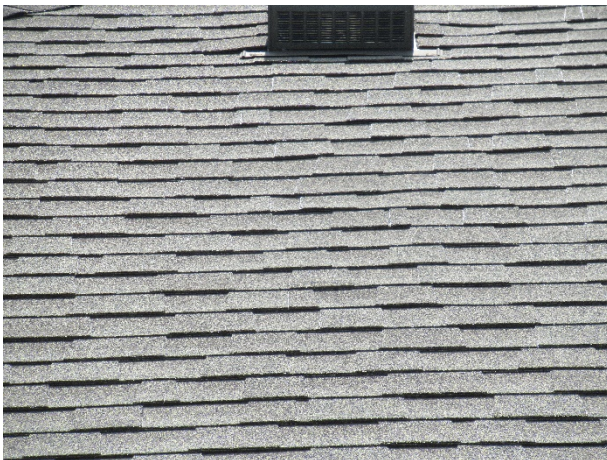
Apparent exposed fiberglass, shown at Building 1
