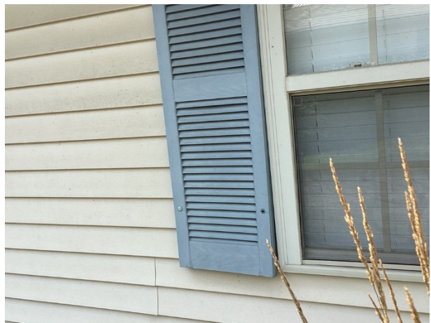
Finish fade and deflection, shown at Unit 182
