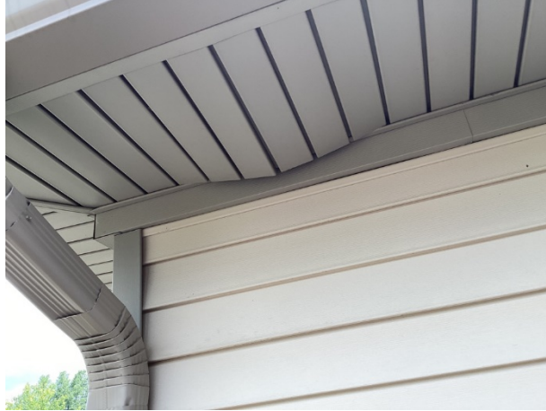
Soffit deflection, shown at Unit 102
