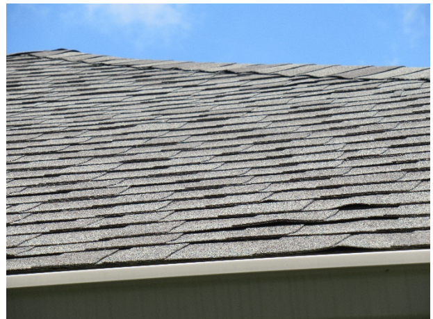
Shingle lift, shown at Building 6
