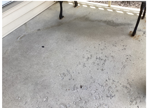
Concrete spall at mailbox enclosure
