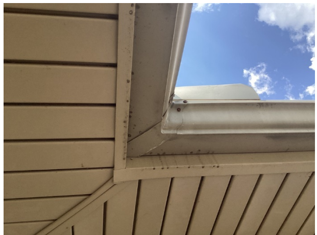
Evidence of water infiltration, shown at Unit 174
