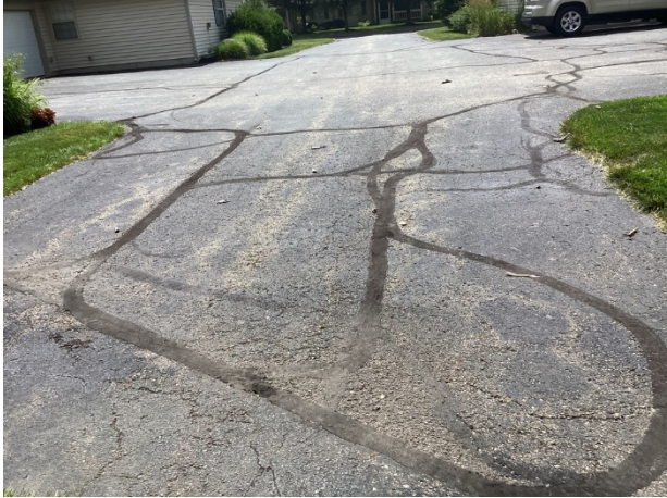
Phase One access drive overview, note settlement and surface deterioration
