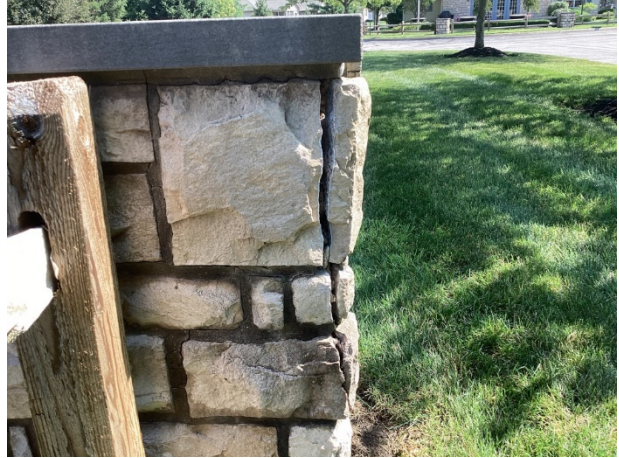
Significant masonry crack
