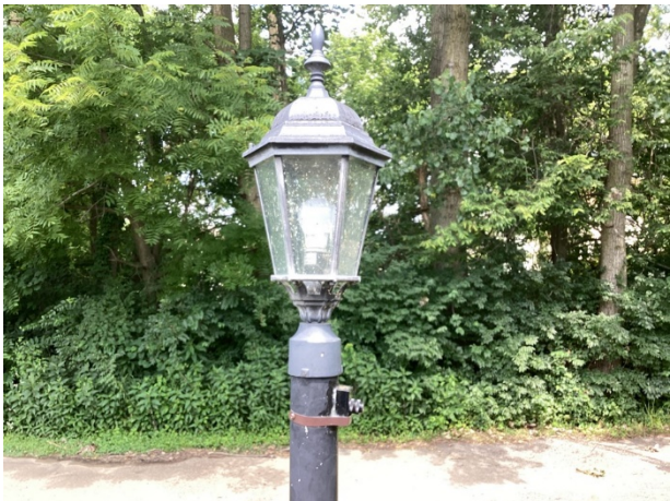
Finish fade and fastener rust
