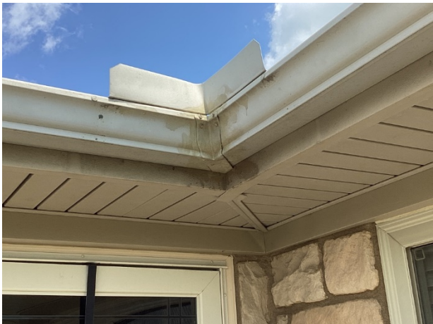
Evidence of leakage at seams
