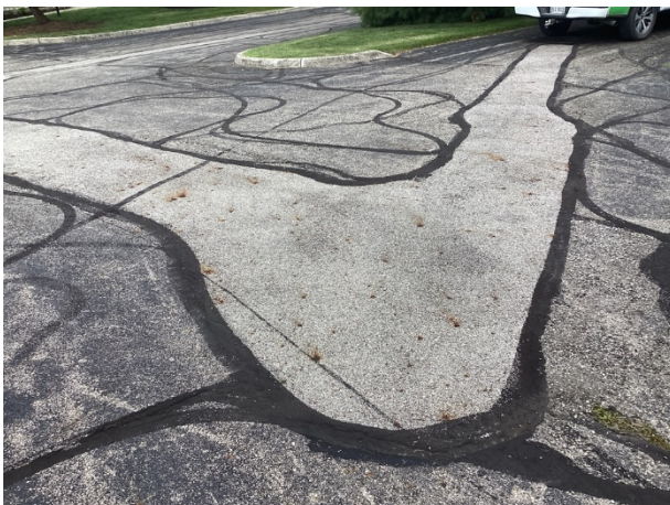
Previous patching and surface deterioration
