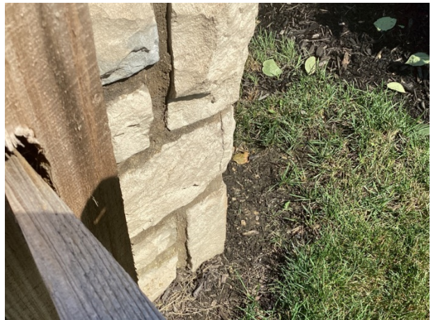
Masonry crack
