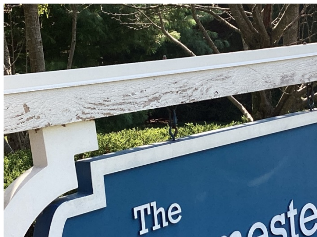
Paint finish deterioration
