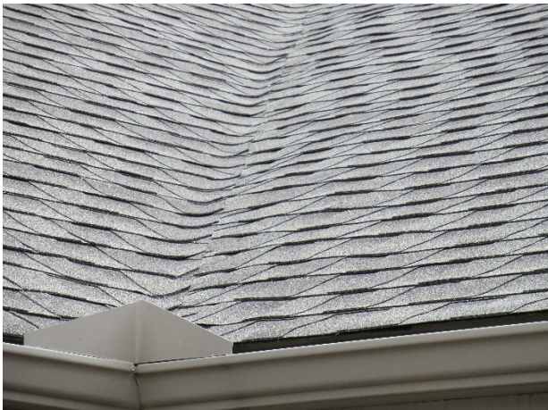
Minor sheathing deflection, shown at Building 19
