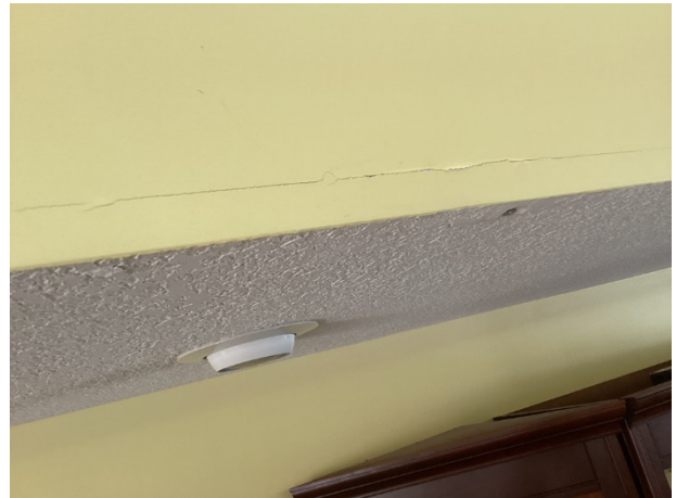
Finish crack
