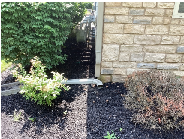
Detached downspout extension, shown at Unit 176
