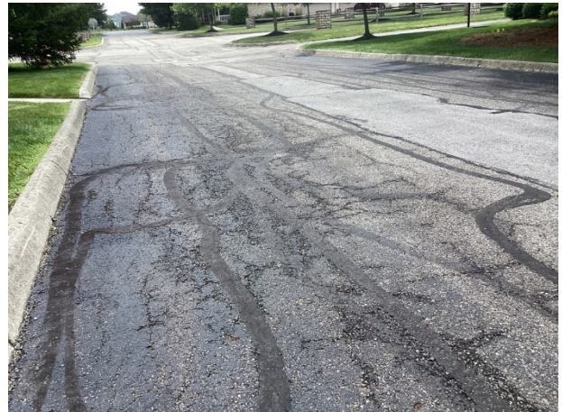
Surface deterioration and previous repairs
