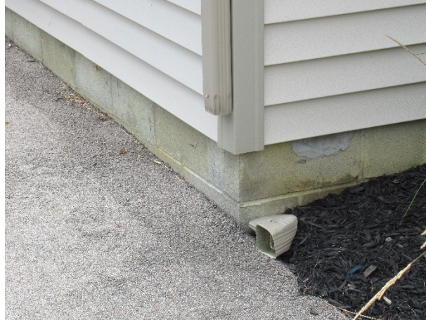
Detached downspout extension, show at Unit 138
