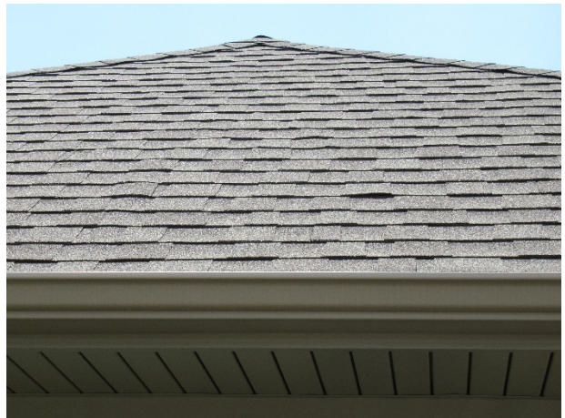
Shingle lift, shown at Building 20
