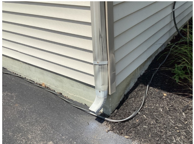
Downspout dents and fastener rust, shown at Unit 184
