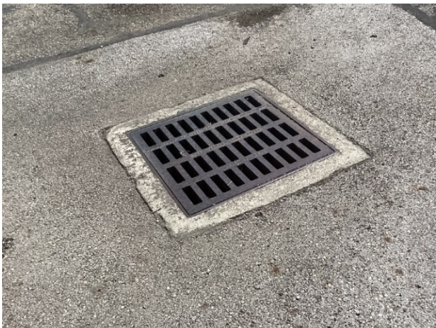
Catch basin, note deterioration
