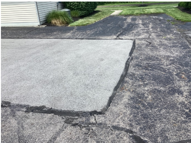
Settlement and previous patching at Phase Two access drive
