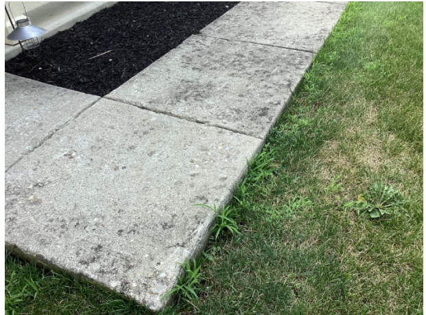
Concrete disintegration, shown by Unit 166
