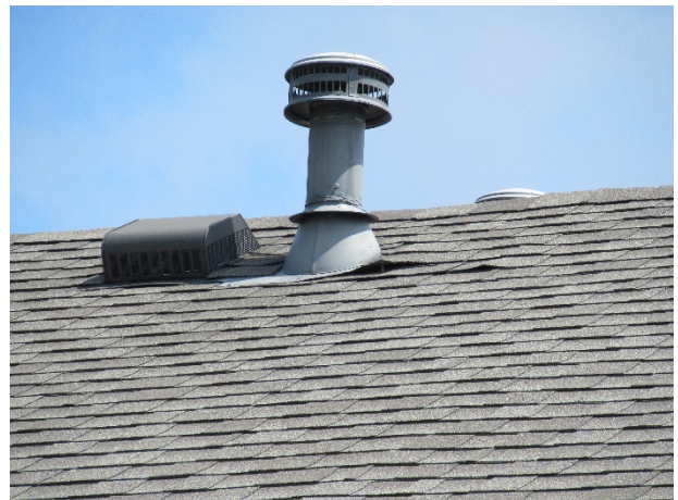
Shingle lift, shown at Building 4
